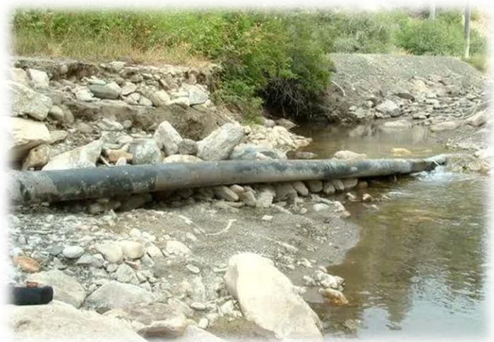
Figure5: Exposed oil pipeline on Beaver Creek near Helena. ( http://ravallirepublic.com )
