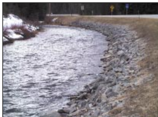
A well designed rip-rap job has 2:1 slopes and does not encroach on the river. This bank could probably have been stabilized using geotextile and vegetative methods with equal success.
