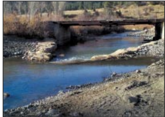
This crossvane weir is designed to control width-to-depth ratio alignment at a bridge cross section.
