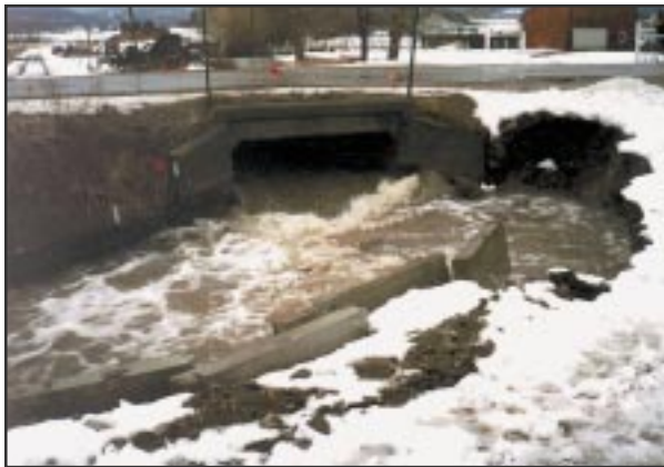
Rigid structures such as median barriers rarely afford long-term success for bank stabilization.
