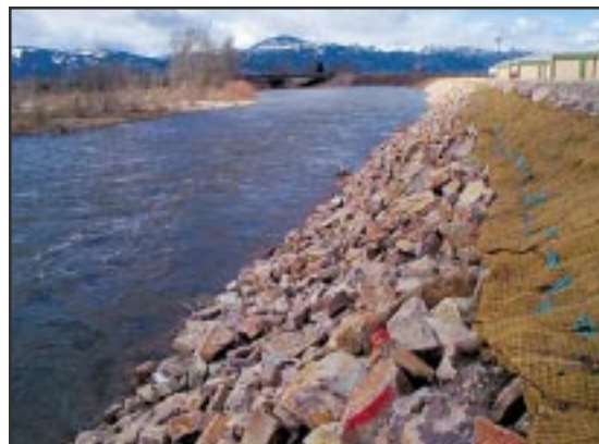
An engineered rip-rap bank provides a high degree of protection, but diminishes natural river values.
