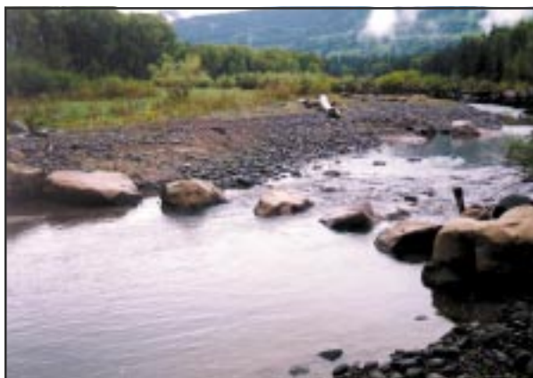
True “V” weirs generally have a row of cap rocks with spaces, rather than a flat sill. This promotes bedload passage (to some extent), but does not always work well for irrigation diversion needs.
