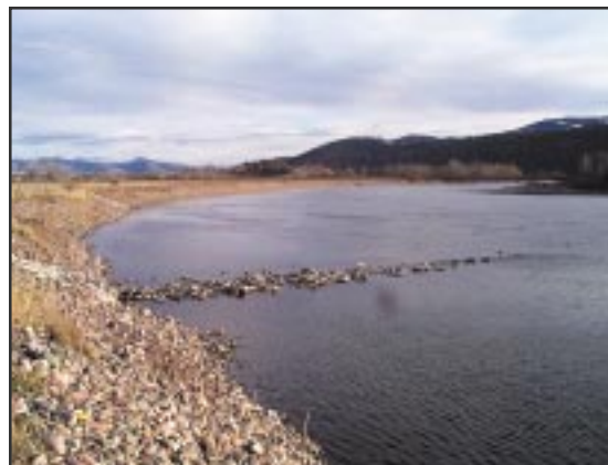
A bendway weir has a gradually sloping profile which shifts the main channel of the river to the outside of the structure. Peak flows continue to use the channel cross section above the weir elevation.
