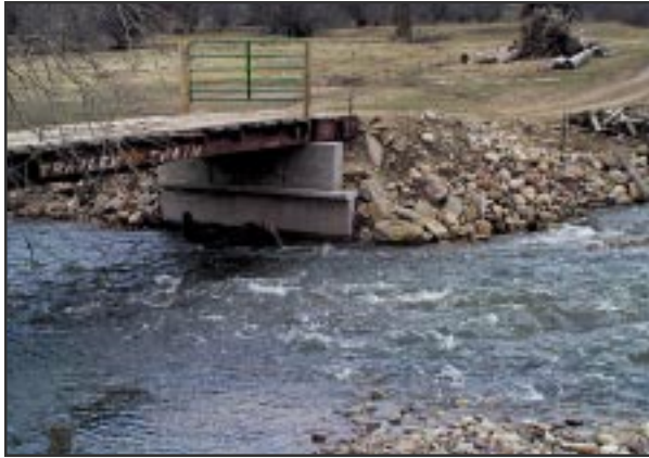
Median barriers don't usually make very good bridge abutments, or retaining walls.
