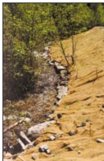
This bank treatment has a rip-rap toe but uses geotextile for the bank and is a good compromise solution.
