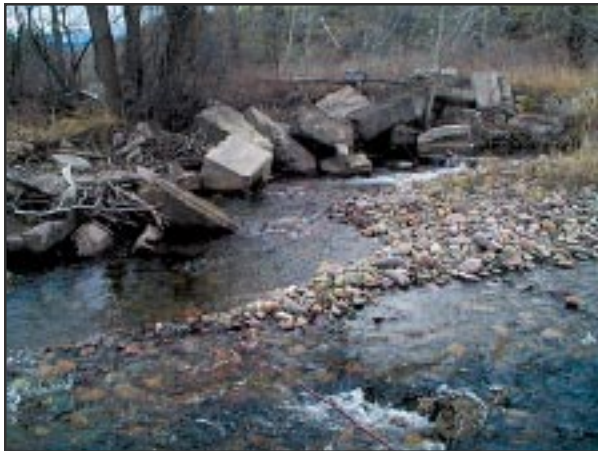
Concrete is generally not acceptable for rip-rap.
