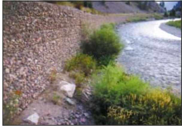
An engineered gabion wall with a rock toe prevents abrasion of wire and undercutting of the footing.
