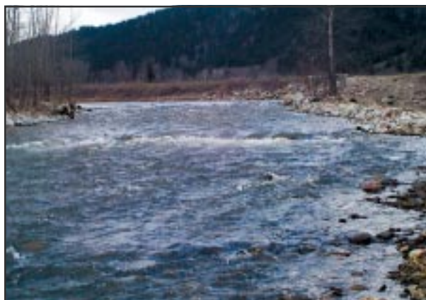
Large weirs must frequently be built in series to avoid large drops exceeding structural stability. Construction of weirs in high bedload transport streams always carries some risk of failure.
