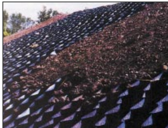
A cellular confinement system can be effective for steep slope stabilization and revegetation.
