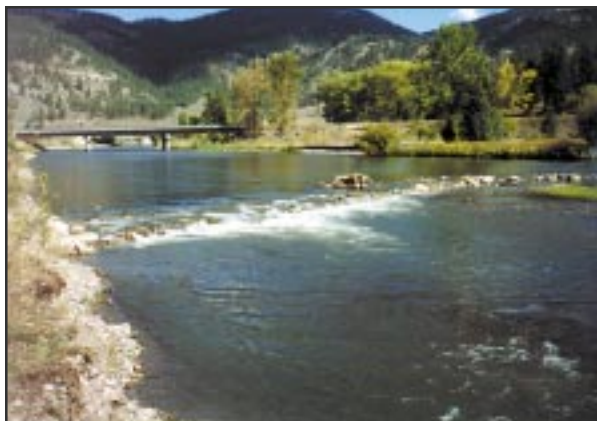
The same structure at left, prior to failure. The warning signs were apparent, notably the elevation of apex above the bed, and 2ft + high drop over the flat sill.
