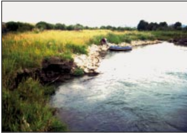
Receding bank upstream of a rip-rap job will eventually lead to failure.
