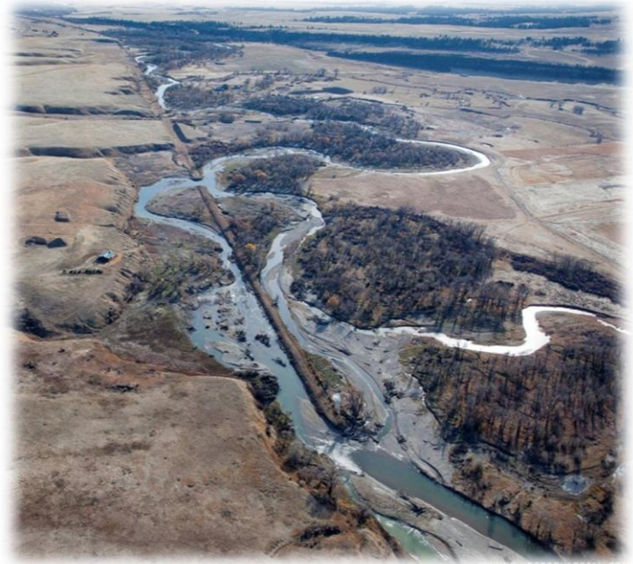
Figure 1. View to east of railroad dike breached during 2011 flood.
