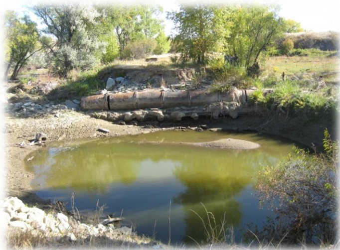
Figure 9. Railroad berm breach where flows overtopped from the backside of the berm.
