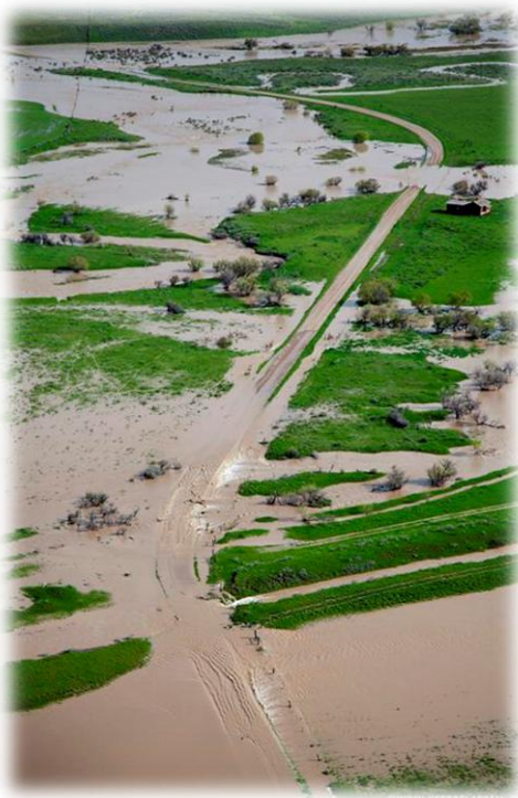
Figure 4. Road prism forming floodplain dike/dam during 2011 flood.
